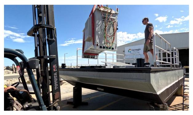
Image: Placement of control system on MoorPower barge prior to PTO unit mounting.
